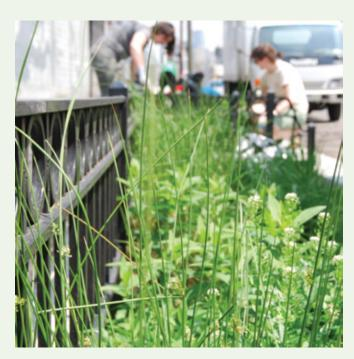
The GCC bioswales are part of a DEP plan to manage stormwater and sewage overflow in the Gowanus sewer shed.
