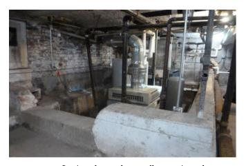
Dry component floodproofing is often an effective solution for equipment that cannot be elevated or relocated out of basements.
