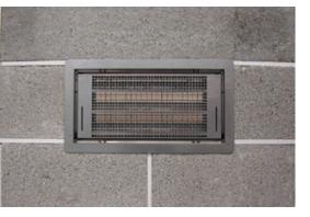
Wet floodproofing vents should be located below the BFE and no more than 1 ft. above the ground.
