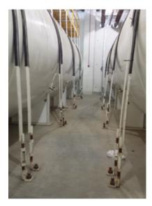
Fuel tanks anchored to a slab. Image: Jon Gravelin.
