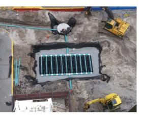
Installation of a stormwater management drywell system. Image: JASA.
