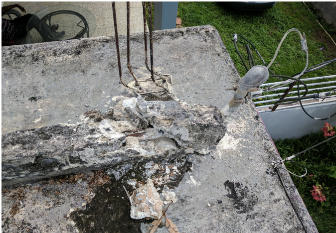
Failed foundation due to inappropriate concrete mix
