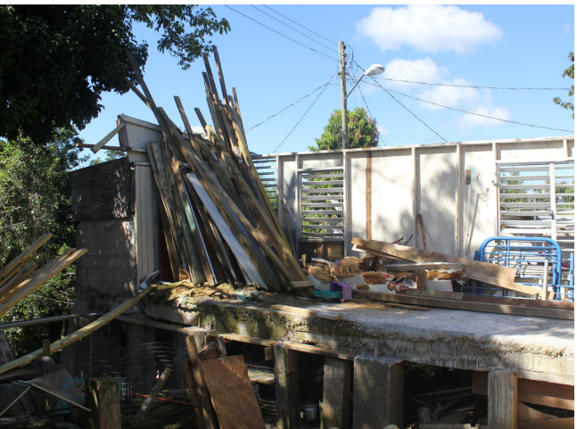
FAILED WOOD ROOF
