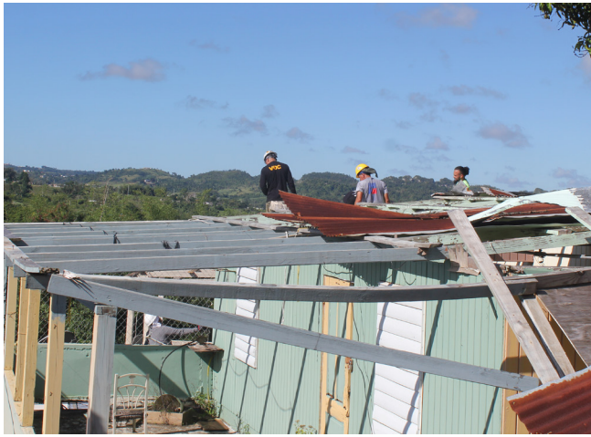
FAILED WOOD ROOF
