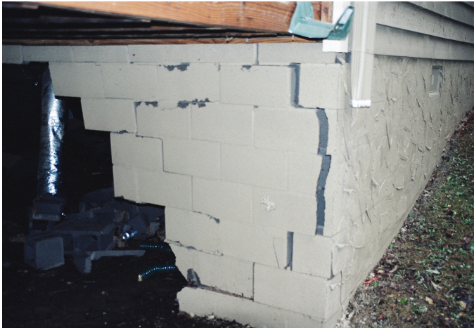
Cracked Foundation
