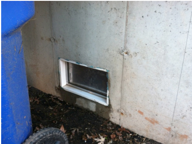
FAILED OPENING = INAPPROPRIATE ANCHORAGE
