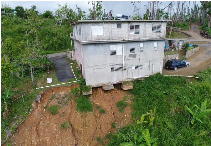
Failed foundation due to inappropriate soil
