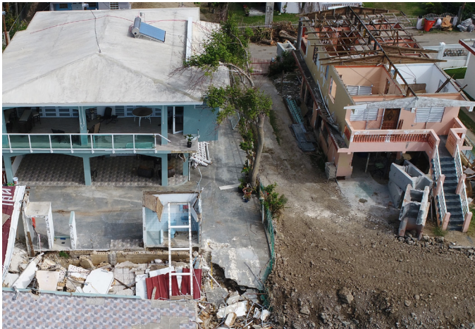
Failed foundation due to weak structural connections
