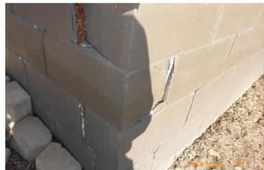
2. Seal all cracks and openings (except for flood vents or openings) below the DFE.
