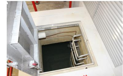
9. Install waterproof hatch doors on sidewalk hatches.
