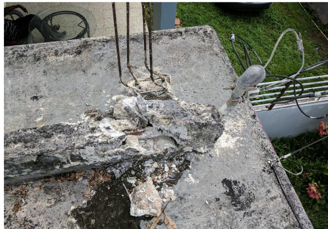
Failed foundation due to inappropriate concrete mix
