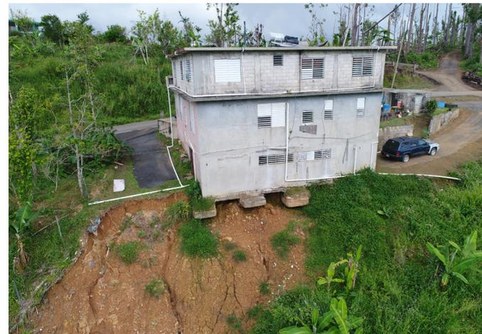
Failed foundation due to inappropriate soil
