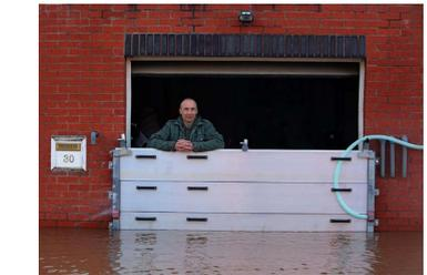
8. Permanently replace first floor doors with flood doors and install removable flood gates over entryways.
