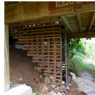
Round or square structures made of concrete or wood embedded in the ground.
