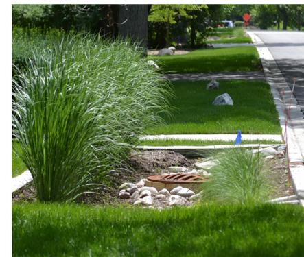
Use sewers or dry wells to collect excess runoff/rainwater. Avoid draining on hillsides and cut/filled areas to minimize erosion. For more info on siting and surface stormwater management, go to Strategy 01: Reinforce Site.
