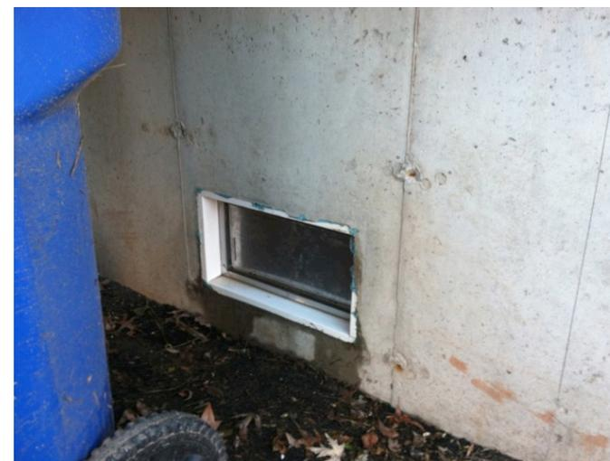
FAILED OPENING = INAPPROPRIATE ANCHORAGE
