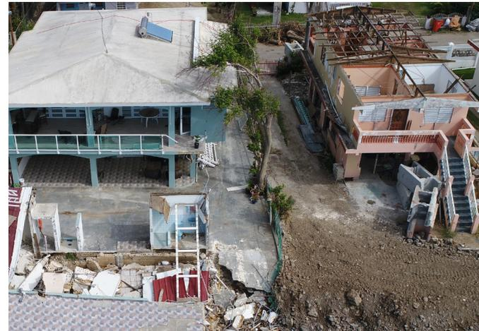
Failed foundation due to weak structural connections
