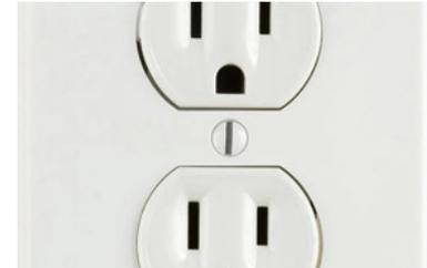
10. All power sockets must be at least 18 in above the floor or projected flood level. Prevent damage to the circuits from flood water.
