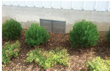
3. INSTALL FLOOD VENTS AND/OR FLOOD OPENINGS IN WALLS
